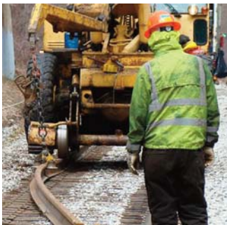
Installation of American-made steel rails
